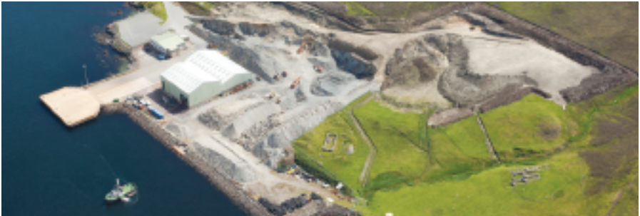
Expansion of lay-down area at Dales Voe.
