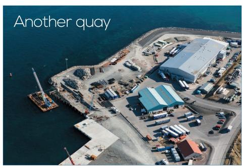
A 75-metre, deep-water extension to Berth 7 at Greenhead Base is on target for completion in October this year and will bring the total quay length in the immediate area to over 780 metres. The site was predredged to nine metres' water depth.
