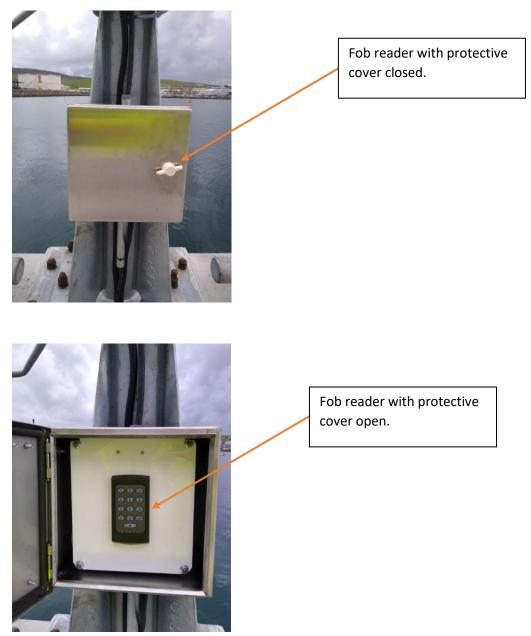
Once activated via fob, the crane will remain powered up for 20 minutes, or until the fob reader is "Double fobbed". To deactivate the crane, present your fob to the fob reader twice, in quick succession.
